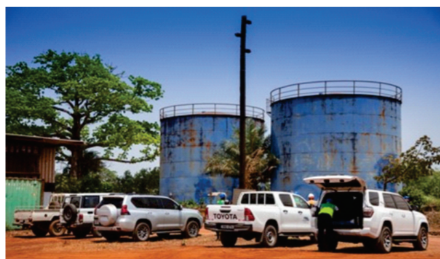
PETROLEUM STORAGE TANKS AT PEPEL
